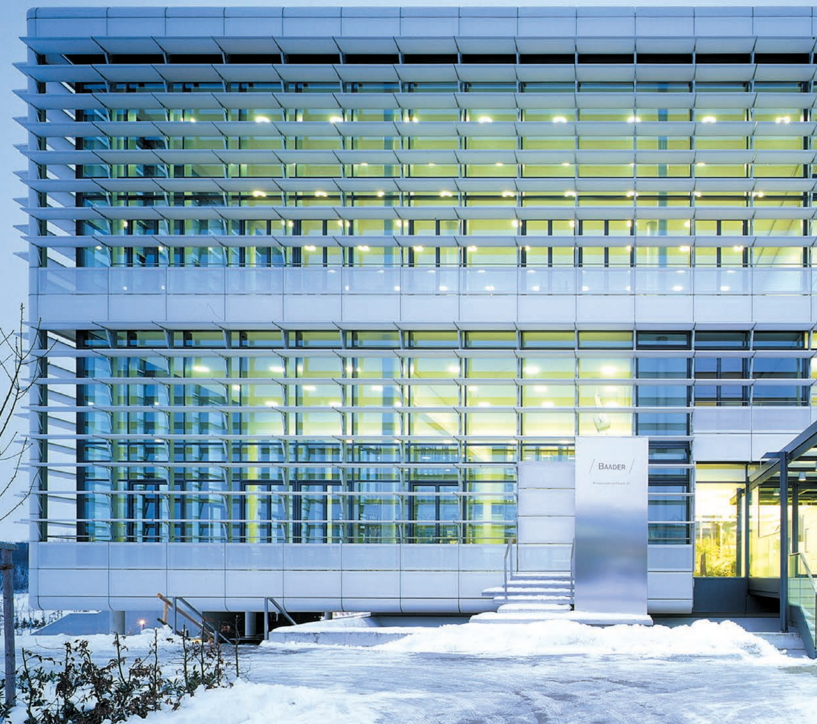
Baader Securities Bank, Munich, Germany. The building has been nearly entirely wrapped in louvres made of PTFE glass fibre Shadotex textile louvres. Louvres are individually adjustable and have greatly reduced the energy use of the building.
