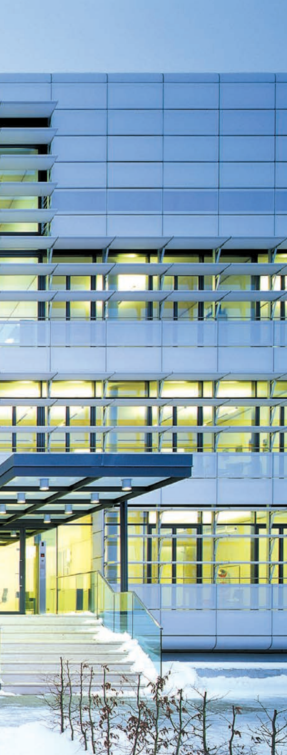
Schwenninger BKK, Germany. The solar shading comprises aluminium tubes arranged in front of the windows giving the building the appearance of a forest or a sugar cane plantation.
