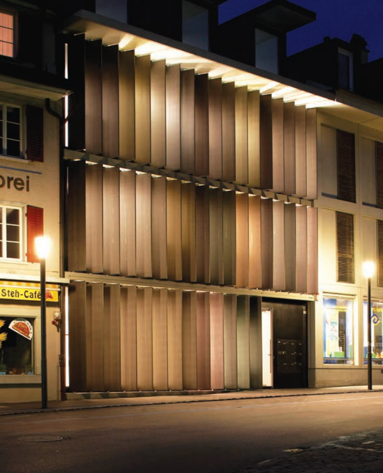
Willi-Beck Bakery, Switzerland. These louvres are installed from ground level up to the eaves and are made from spruce and fir, giving the building a unique character. The wood has a dark grey coloured iron oxide paint applied to them, which enables their appearance to change depending on the angle at which they are opened.
