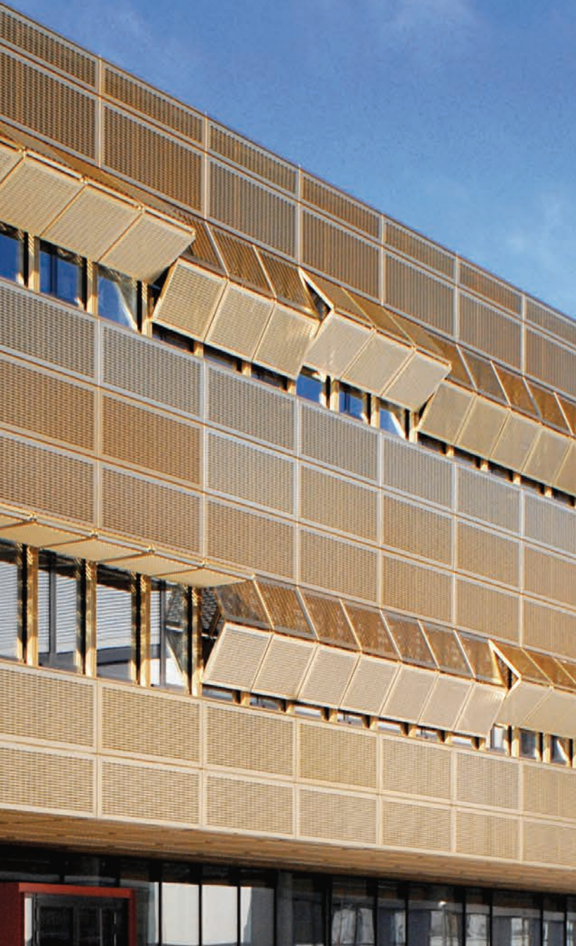
University of Potsdam, Germany. Gold anodised vertically folding shutters which open and closed according to the position of the sun.
