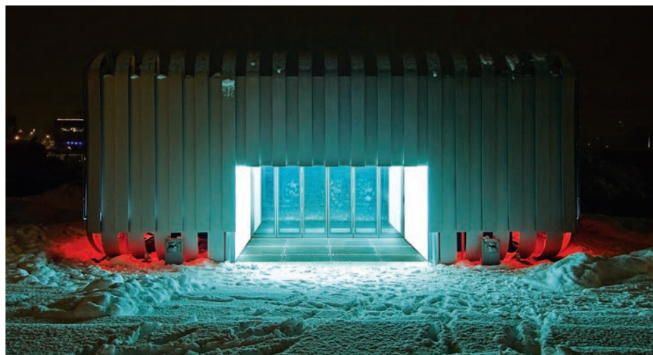
iHomeLab, Switzerland. The louvres give an appearance of a fish moving. The louvres themselves consist of a total of 380 fixed and 300 moveable louvres installed vertically on a building which has an exceptionally high thermal performance.
