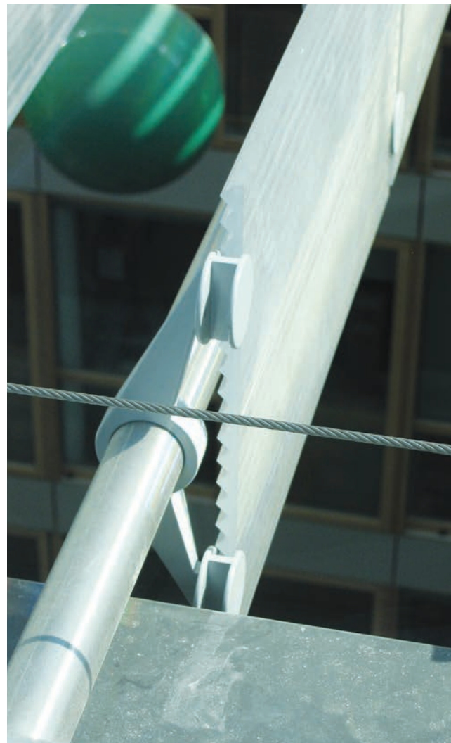
This shows a detail of the structure of a prism louvre. The louvres themselves are made from highly transparent PMMA plexi-glass, which is UV and weather resistant.
