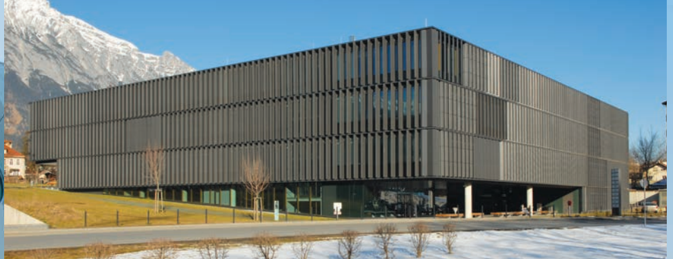
Tilak Competence Centre, Innsbruck, Austria. 964 moveable louvres comprising an area of 2925m 2 of solar shaded façade.
