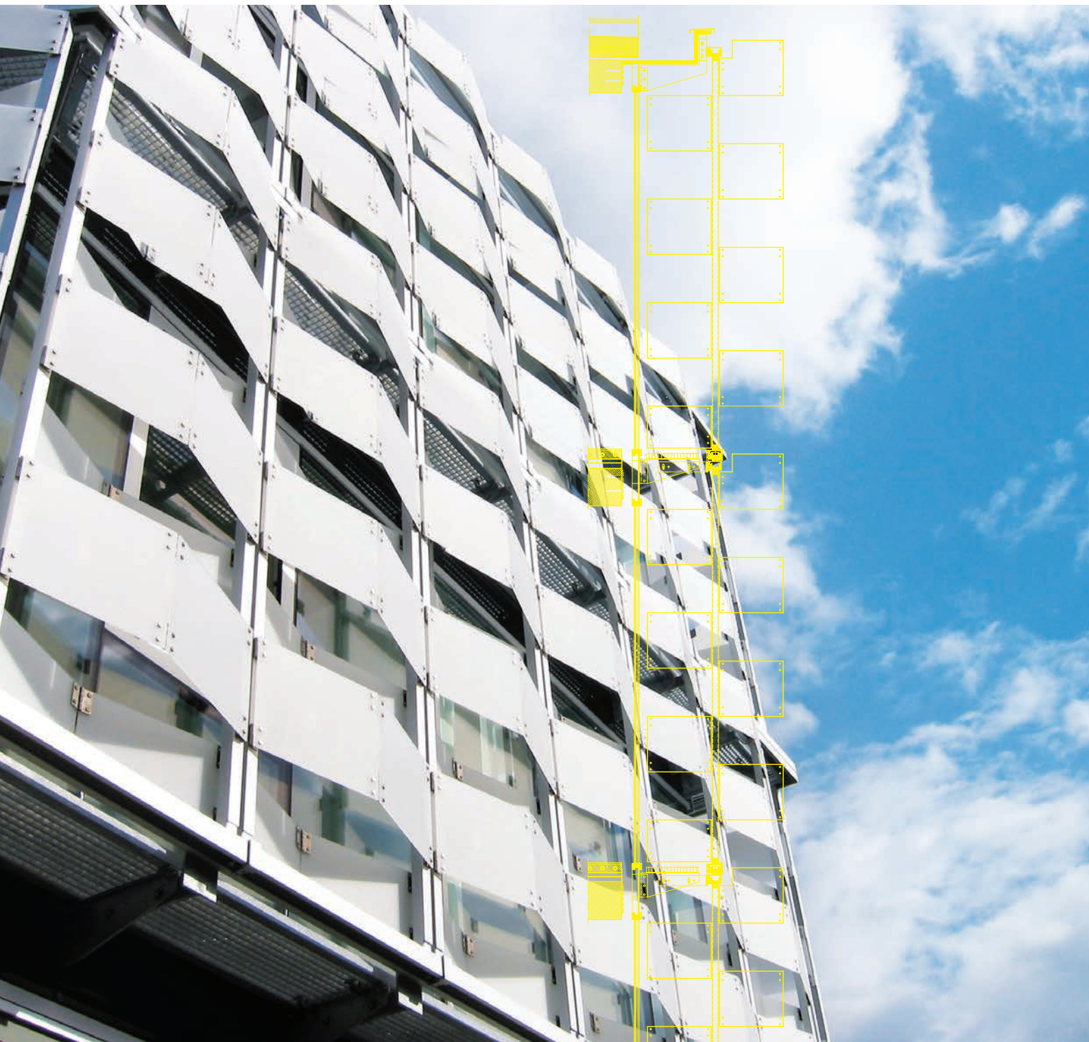
Milsertor House, in Hall, Austria. Plexiglass folding shutters provide an appearance of flags hanging off the building, whilst providing excellent solar shading and good outward vision.
