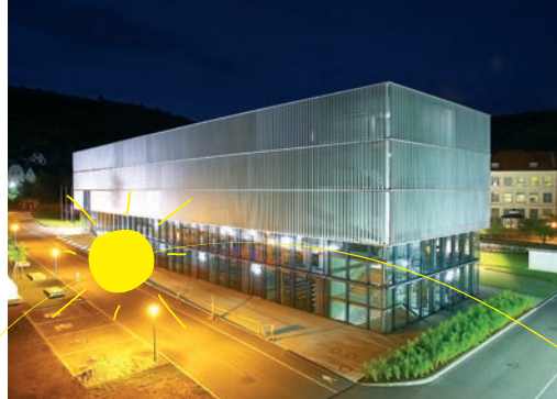
Campus Krems, Austria. Moveable fabricated Shadometal louvres are 25% perforated and cover the complete façade in two elevations. At night the louvres are fully opened in order to provide night cooling. At 4 o'clock in the morning the louvres close to ensure that the complete building is shaded. In winter time the sun's rays passively warm the building and glare is reduced as the louvres track the sun.
