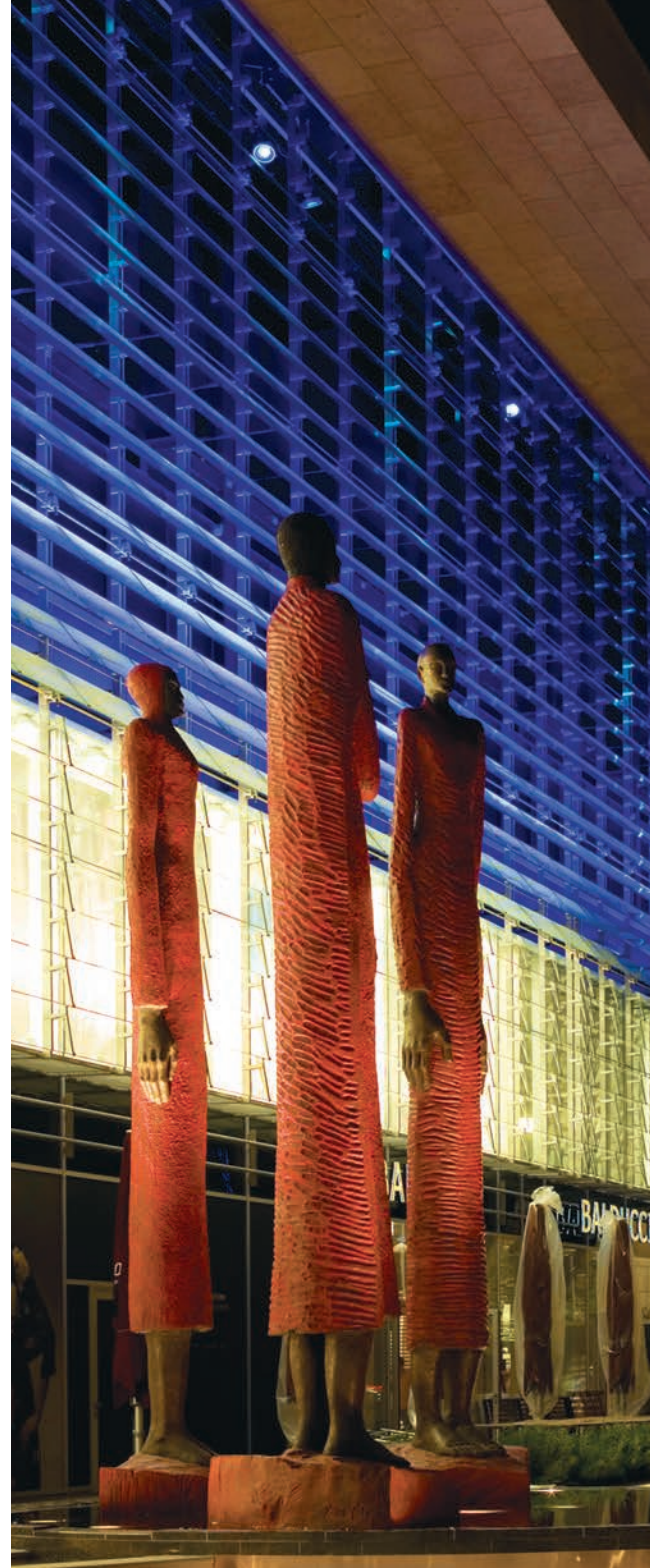
Alstertal Shopping Centre in Hamburg. 809 coloured back-lit adjustable glass louvers emphasize the living character of the urban quarter
