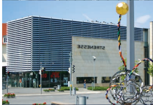
Strenesse store, Metzingen, Germany. Fixed Solarfin solar shading system designed for optimal solar shading.
