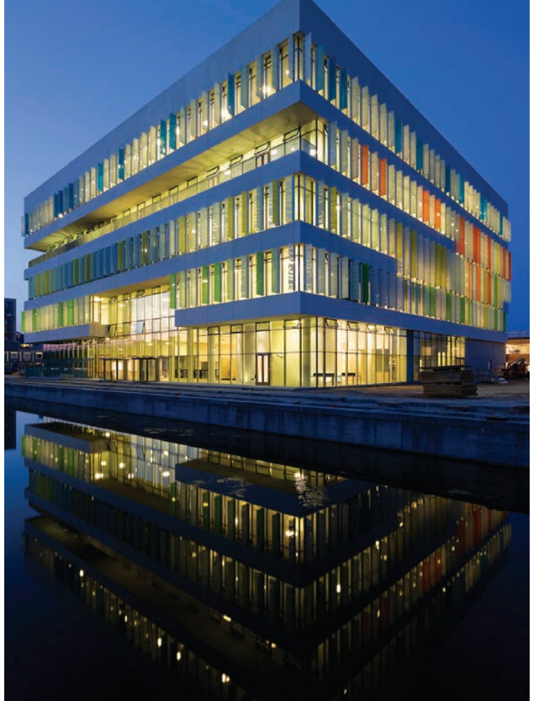
Ørestad Gymnasium, Copenhagen, Denmark. Many of the glass louvres are coloured crating a subtle effect inside the building.
