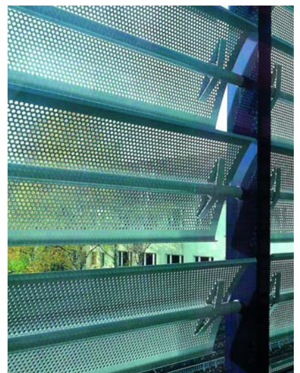
SD Worx, Germany. Controllable perforated Shadometal.
