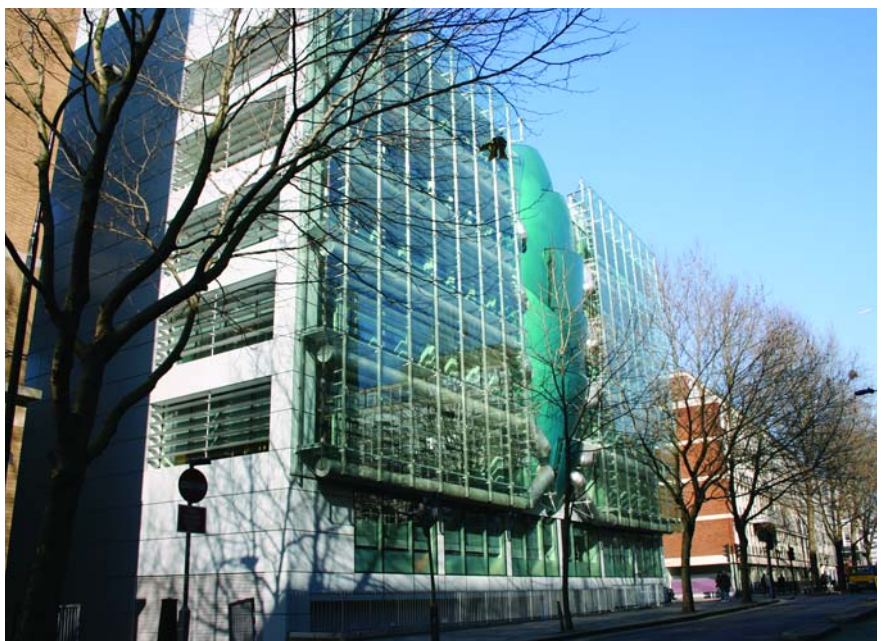
Arup Fitzrovia, London. Fixed Solarfin supported by drop rods, and Universal Louvre fitted to plant rooms.
