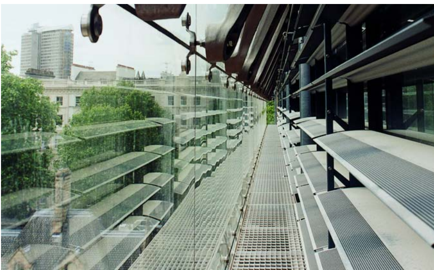
Natural History Museum, London. Between the Colt glass façade and walkway of the stunning South façade is a bespoke, controllable fin, which is half perforated to provide additional daylight when in the closed position
