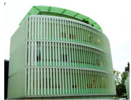
Clear Channel Outdoor, London. Both fixed and movable vertical Solarfin louvres installed onto the facade.
