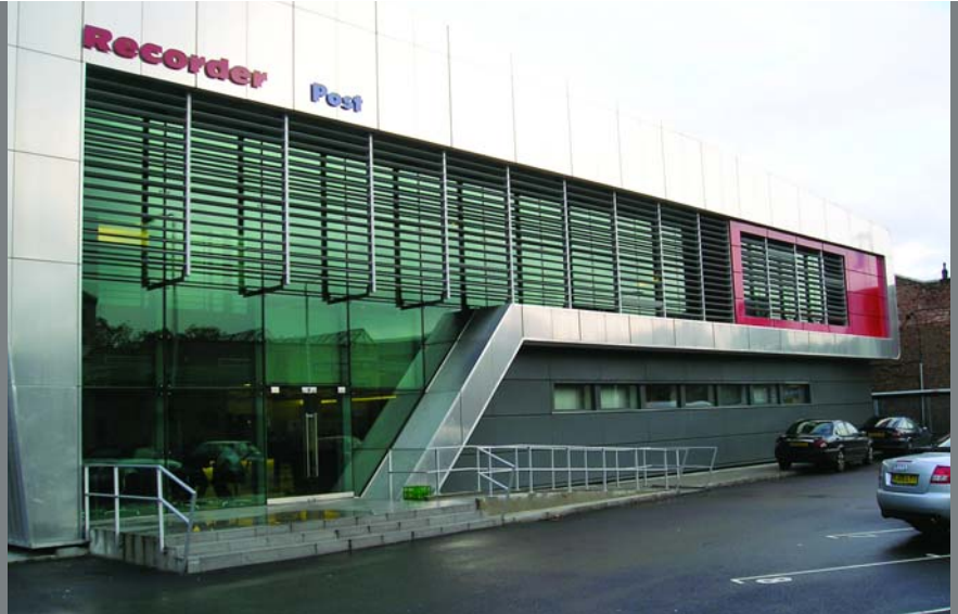
Ilford recorder, Ilford. A series of movable Solarfin louvres were integrated into a "PIA" mullion-integrated actuation system consisting of box section mullions with hidden mechanisms inside, controlled by a Colt ICS 4-Link control system.
